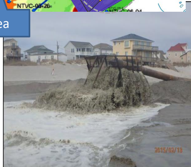
Figure 35. Rock box installed during dredging operations.
